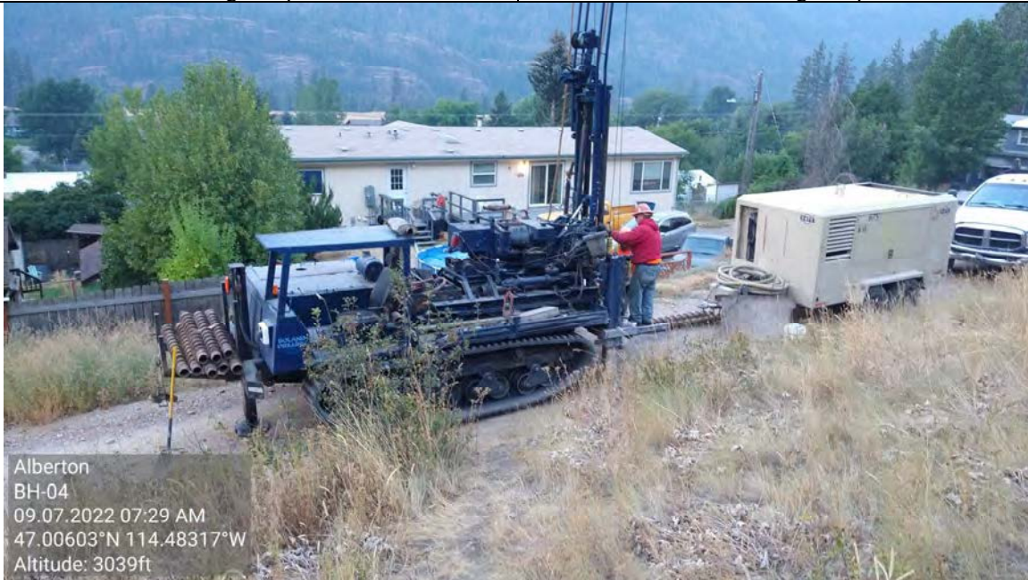
Picture # 3: BH-04 Drill Rig Setup
