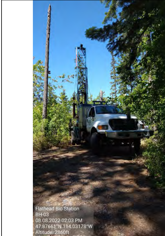
Picture # 19: BH-03 Drill Rig Setup
