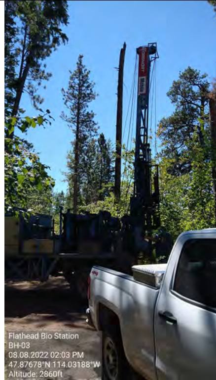
Picture # 20: BH-03 Drill Rig Setup
