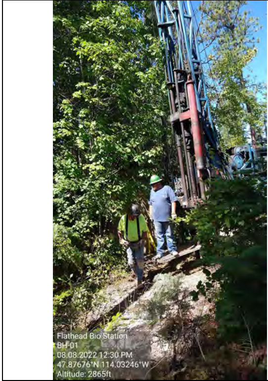
Picture # 3: BH-01 Drill Rig Setup
