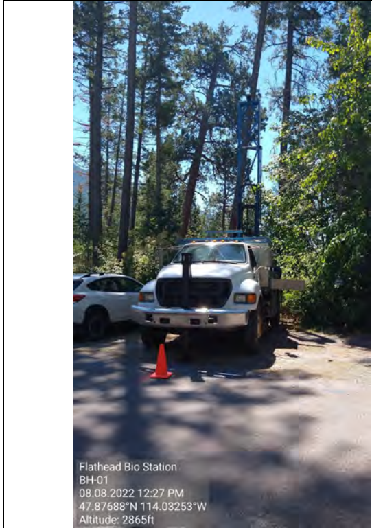
Picture # 1: BH-01 Drill Rig Setup
