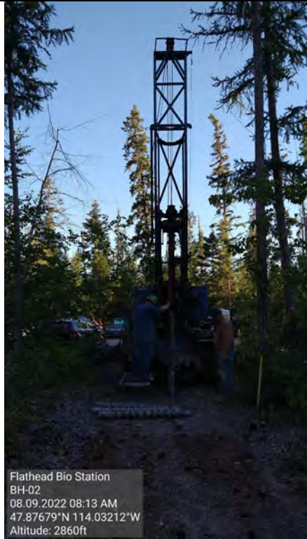
Picture # 10: BH-02 Drill Rig Setup
