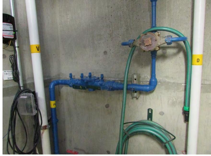
There is an RPZA in place at the wastewater treatment plant for cross connection protection, above right.
