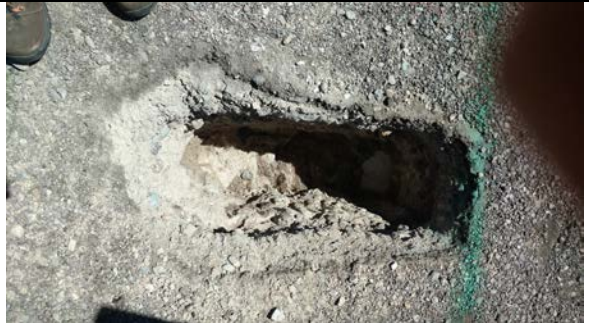
Picture # 2: BH-01. Utility locate "pothole".
